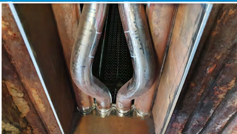
RWE Huckingen power station TÜV programme Boiler pressure part and replacement of the fuel injection cooler 16Mo3, 13CrMo4-5, 10CrMo9-10 5,000 hours September - October 2019
