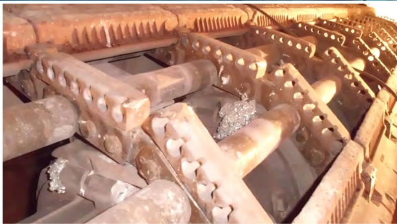
Boehringer Ingelheim Pharma GmbH & Co.KG Combustion grate boiler 8 Delivery of spare parts, execution of inspection work on the travelling grate, build-up welding 2015 - 2018
